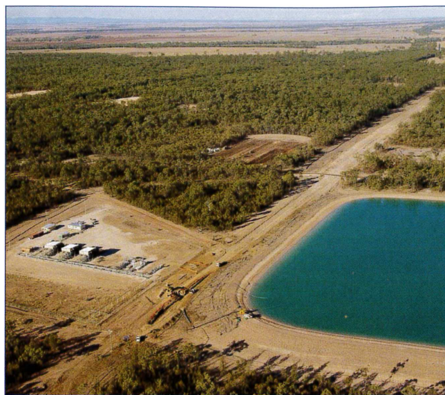
A typical dam and gas extraction facility. See page 71.
